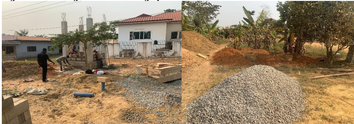
Figure 17: Drilling and mechanising of boreholes
