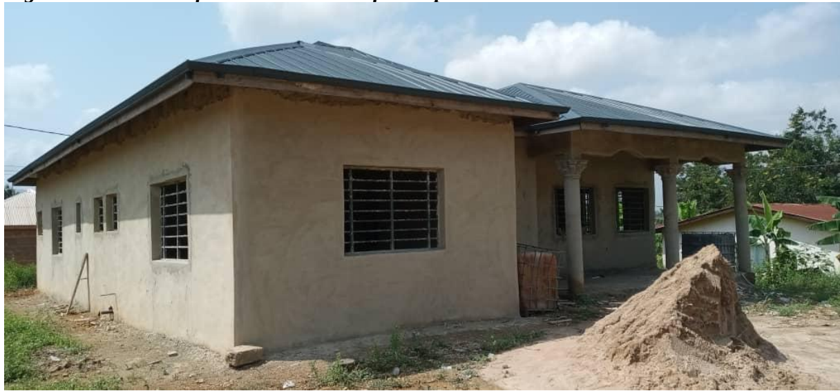
Figure 16: Picture of the construction of 1No. police station
