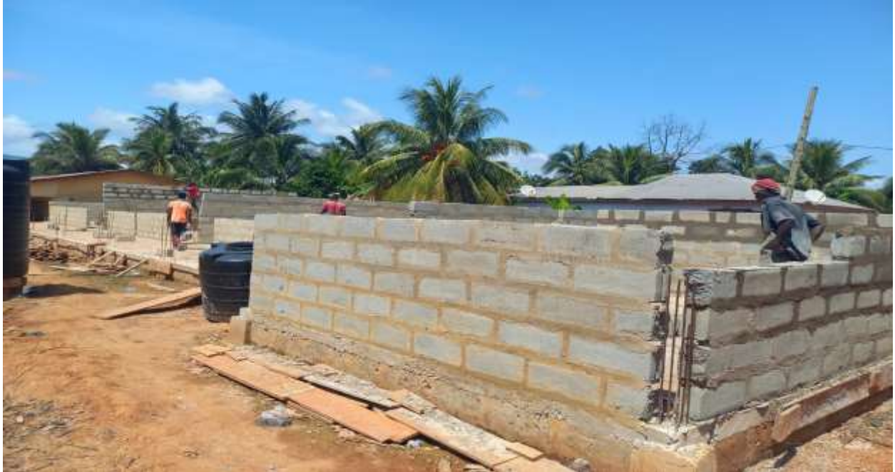
Nsutam SDA JHS Block under construction
