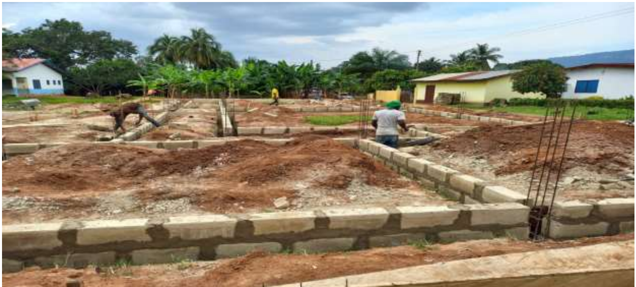
Hemang SDA JHS Block under construction
